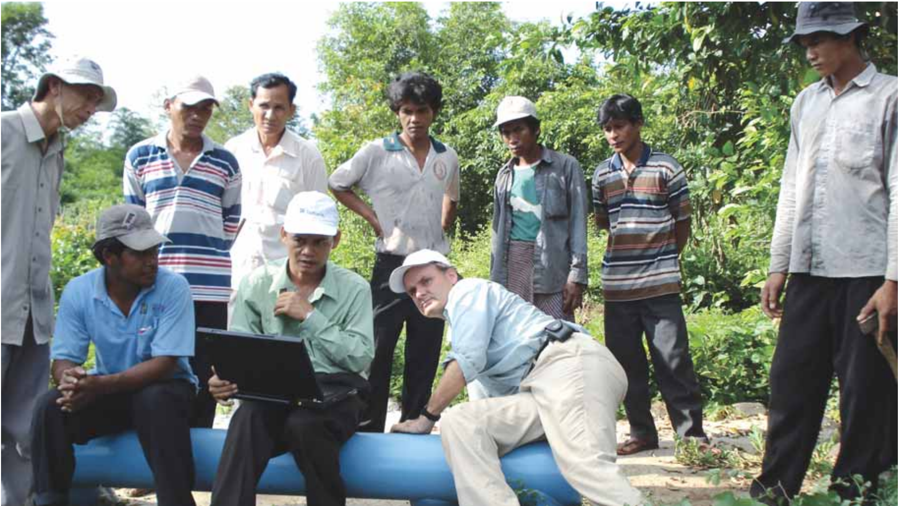
Toni and his team check the calculations in his electronic bridges system before hanging cables.
