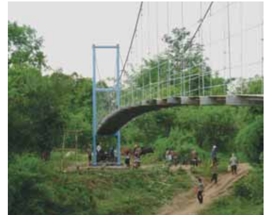
Markets and activity flourish around the new bridges.
