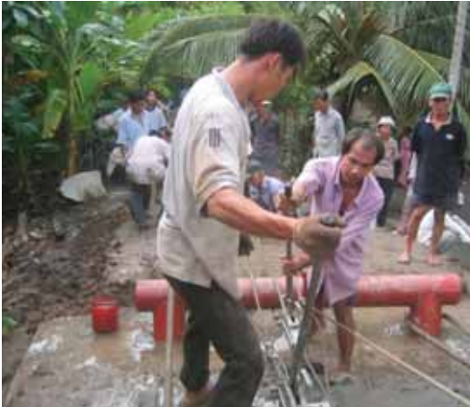
Villagers work together to construct their community bridge.
