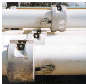
▲ Coated line pipe with installed anode using anode pads
