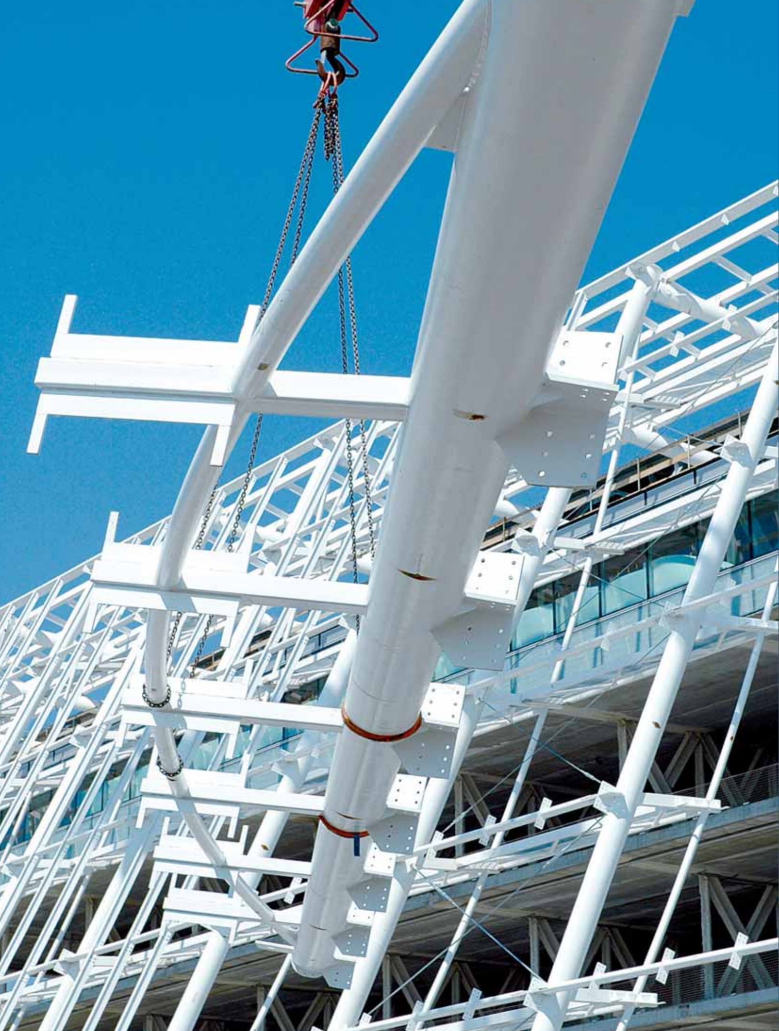
The New Hospital in Mestre - Italy
