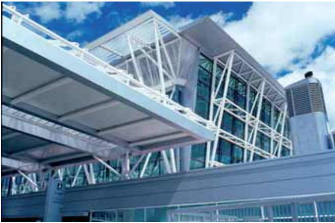
International airport Pizarini, Terminal A , Buenos Aires, Argentina / Canopy roof
