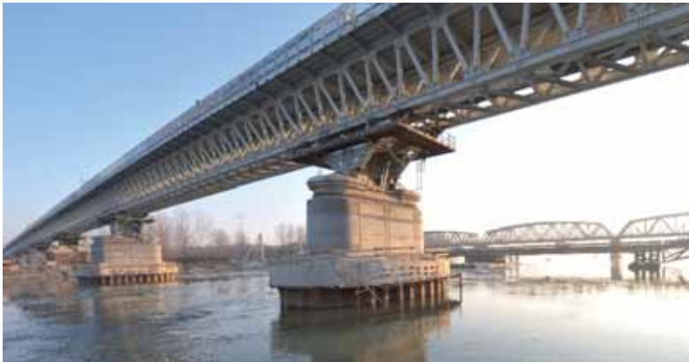
Bridge on the Po river, Piacenza, Italy / Tubular steel supporting the bridge
