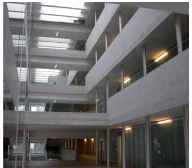
Bocconi University, Milan, Italy / Steel structure to support the roof
