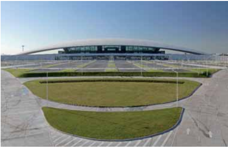
Carrasco International Airport, Montevideo, Uruguay / Supporting structure for roof and glass façade
