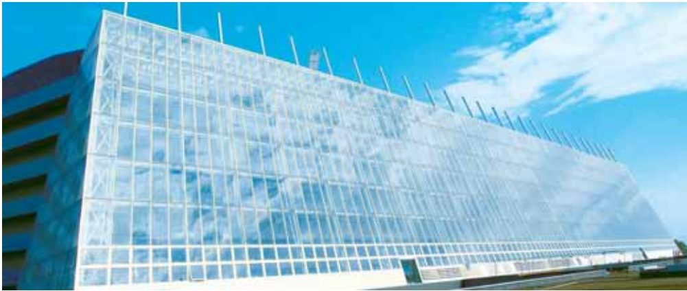
Hospital in Mestre, Venice, Italy / Tubular structure for the "Sail"
